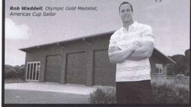
Recently constructed 14 x 16 x 4.2m American Barn with ply & batten cladding on end wall and internal dividing wall. Built near Matamata, this shed utilises a partial clear span design to provide an unobstructed work shop area.
